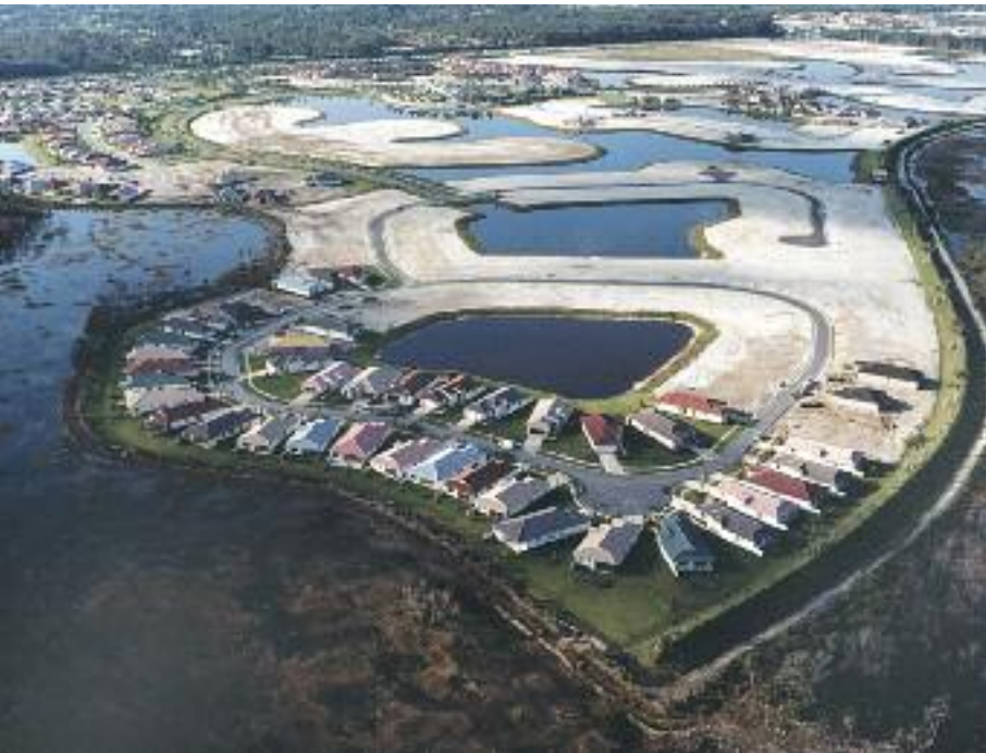
Above: Retention pond excavation for a large-scale residential site development job near Royal Palm Beach, Florida.
