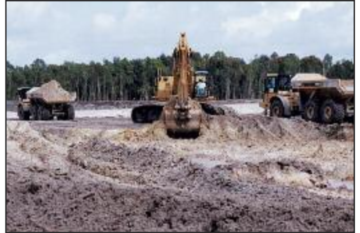
Above: Retention pond excavation for a large-scale residential site development job near Royal Palm Beach, Florida.
