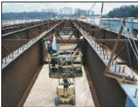
Above: Crew members verify proper torque of bridge bolts on a SR-288 project in Richmond, Virginia.
